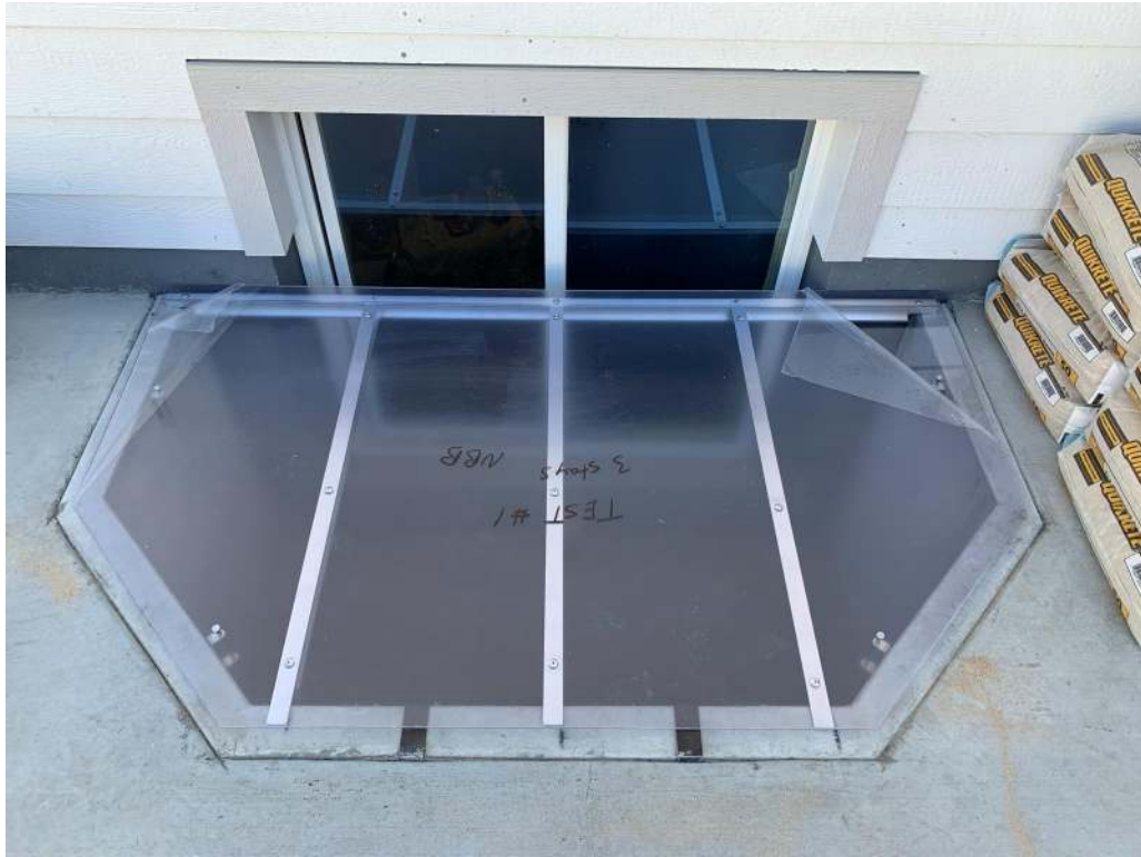
Photograph 2 – Specimen 2 Window Well Cover
